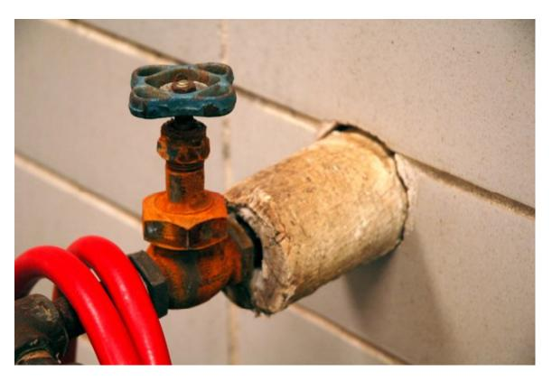
A rusty water spigot with a dirty, cracked insulated pipe. *Lm* could spread to the hose and be sprayed in the establishment.
