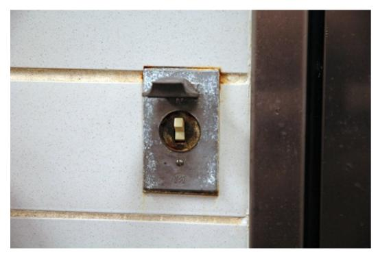
A light switch with residue build-up and grime. The switch could be contaminated with *Lm* by employees' hands during operation, and may not be cleaned during sanitation. When the light is turned on the next day, the hands could be re-contaminated.
